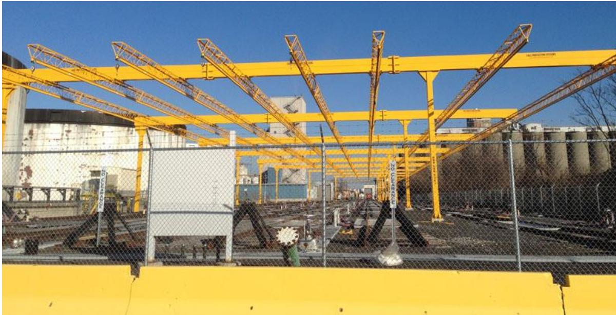
A large company in Albany, New York came to Fall Protection Systems wanting to provide fall protection for their employees. They needed a custom solution and they were looking to cover 8 tracks that contain hopper and tanker cars. FPS custom engineered a system that not only met all of their needs, but one that was the most effective and efficient solution in terms of cost and employee access. This is the largest turnkey project that FPS has ever taken from design to completion.
