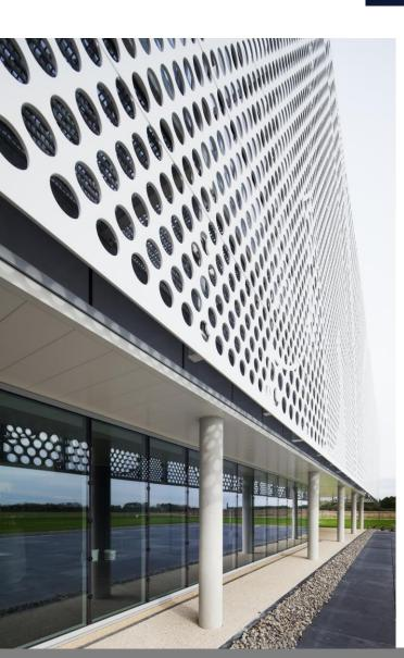
HI-MACS® creates a balance between the project's size and structural system. Also, panels were installed and attached to metal posts making the structure seem light and delicate. For the LCCA fabricator, the main constraint was to hide the fastening systems while allowing for the mechanical stress related to the exhibit. HI-MACS® knew how to meet the expectations of both the client and various service providers.
