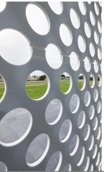
Located in Givrand (Saint-Gilles-Croix-de-Vie area), BENETEAU's (a major sailing boat, yacht and motorboat manufacturer) headquarters has an original façade designed using HI-MACS® new generation acrylic stone. With thermoformable, multipurpose, ultra-resistant and non-porous properties, HI-MACS® proved to be the perfect material for the project.
