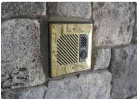
Flush-Mounted 8028 SIP Doorphone using Brass Faceplate
