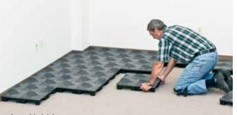
Assembled right over carpet or foam pad for bare floors. No demolition.
