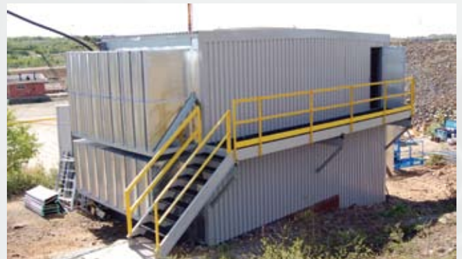
Mine Fan Intake Noise Enclosure
