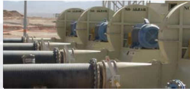
Circular EPDM Rubber Expansion Joints for Mineral Processing Facility in South America
