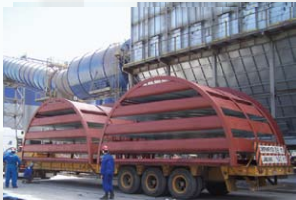
Stack Silencer for South American Power Plant
