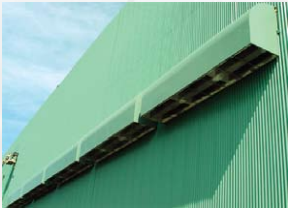
Intake Cowl Silencer for Gas Turbine Building Installation
