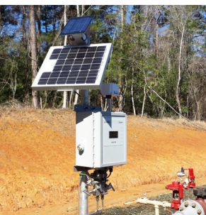
Telemetry monitoring systems for remote production well sites.
