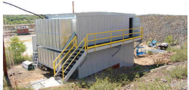
Mine Fan Intake Noise Enclosure
