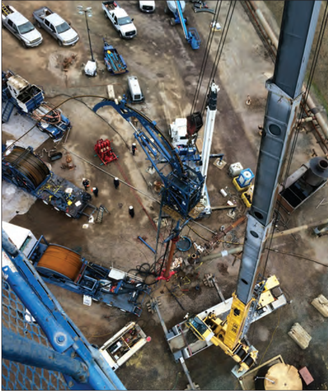
1st Place: Coil Tubing from 125 ft. Manlift by Jay Hepper, Cobb, California, USA.
