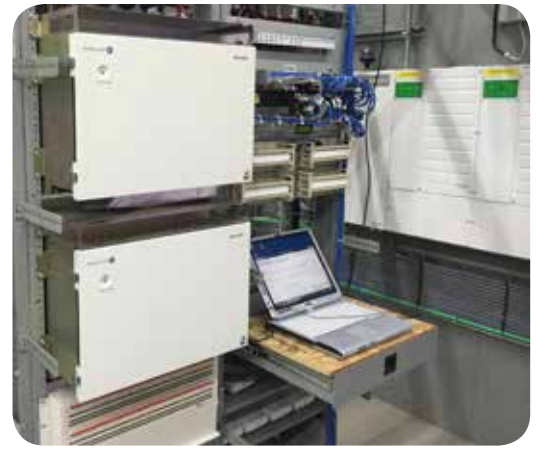
Carrier-grade microwave radios and multiplexers are supported for 24/7 operation by an Iron Edison Lithium Iron 5000Ah 52V battery. Inverters from Schneider Electric (right) provide AC power for other site loads.
