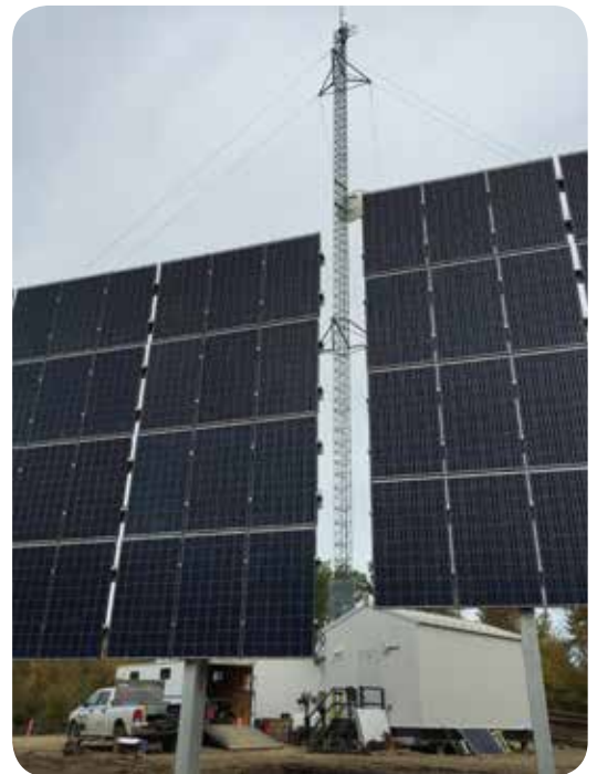
An Iron Edison Lithium Iron battery supports the telecom equipment at this site in Alberta, Canada. The site was converted to all renewable energy, eliminating the need for generators completely.
