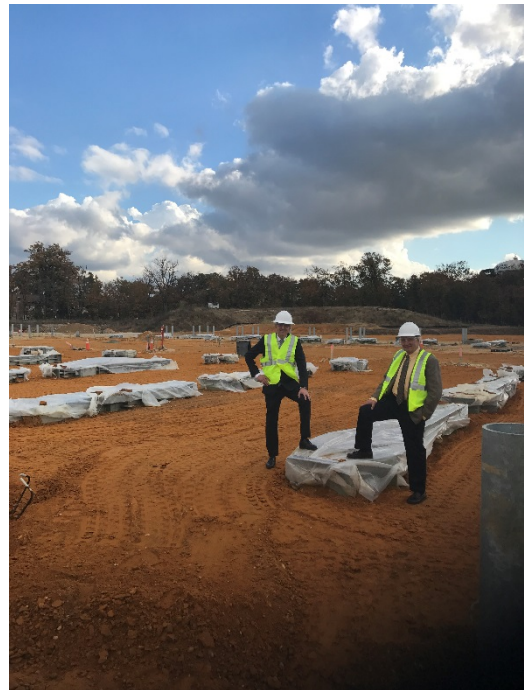
Stertil Group CEO, Ulbe Bijisma (left) and Stertil-Koni USA president, Dr. Jean DellAmore (right) at Washington Metropolitan Area Transit Authority (WMATA) construction site where Stertil-Koni DIAMOND LIFTS are to be installed in new vehicle maintenance facility.
