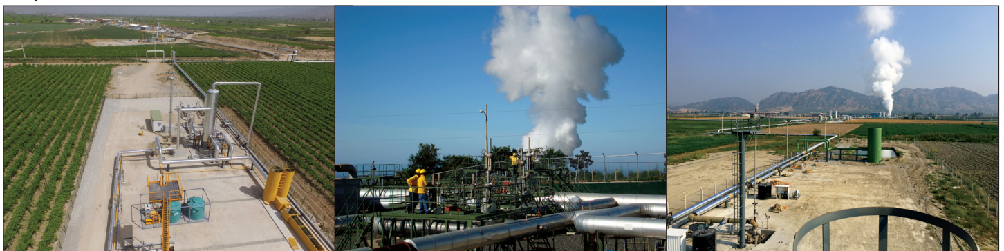
1st Place , Kristi McGinley, Kemaliye Gathering System | 2nd Place , Paul Moya, Commissioning at Las Pailas I | 3rd Place , Kristi McGinley, Efeler 1 Gathering System
