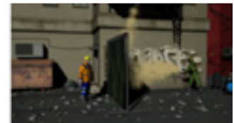
Sandblasting Job Site
