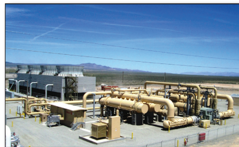
Cyrg Thermo Geothermal Power Plant
