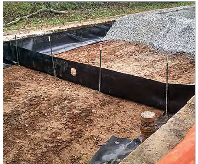
Figure 7. A check dam in place ready to receive supporting aggregate.
