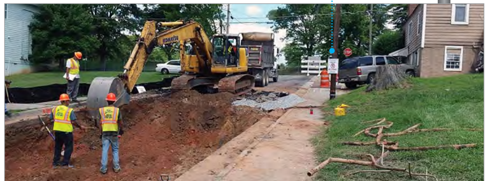
Figure 2. Excavation included removal of abandoned utility lines.
