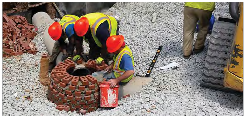
Figure 3. Reconstructing a brick manhole.
