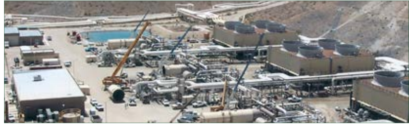
Coso Geothermal Power Plant (Courtesy Coso Operating Company)
