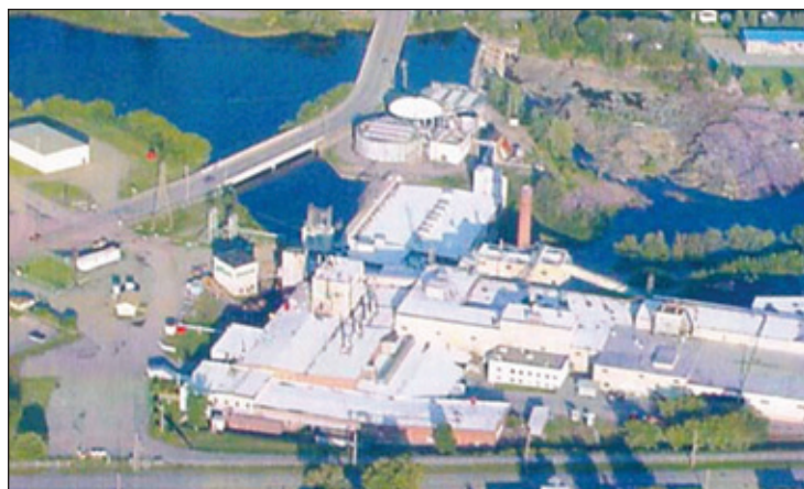
The Weyerhaeuser Pulp & Paper Mill, Sturgeon Falls ON: Extensive Asbestos Abatement, Hazardous Materials Removal, Soil Remediation and Demolition of a 300,000 square foot facility.
