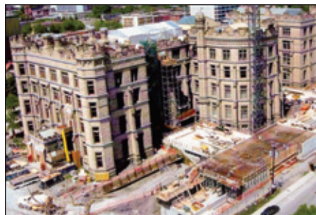
Museum of Nature Ottawa, 2004-2008: Demolition and Abatement Project, Historic Building Site
