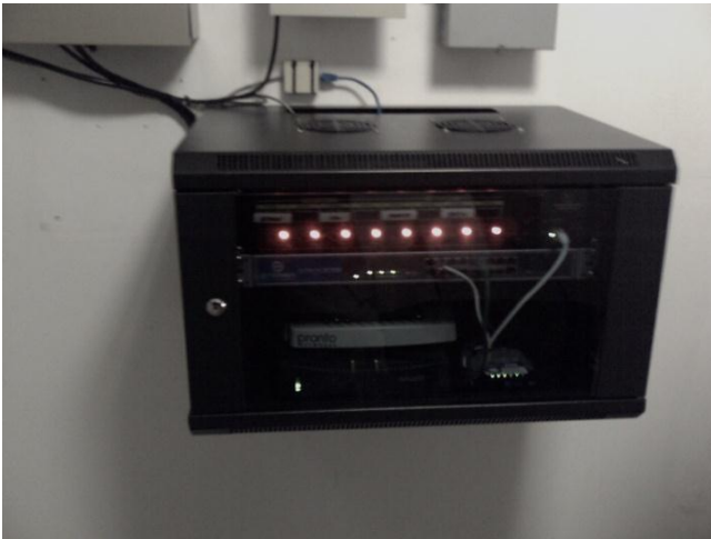
SON Networks' equipment in demarc/telephone closet for medium sized property or common area only deployments.
