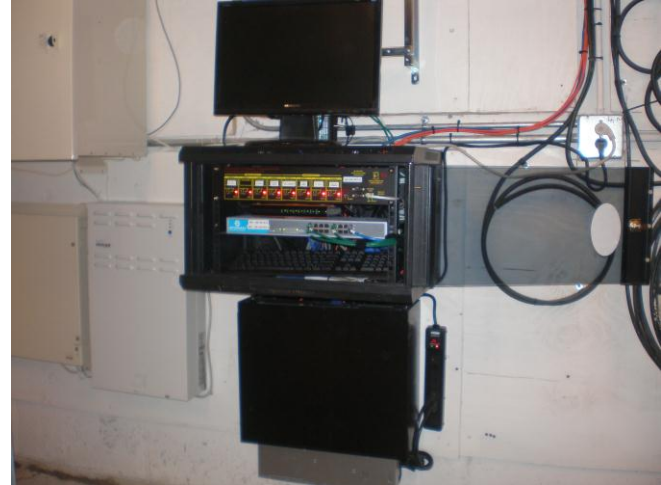
SON Network's equipment in demarc/telephone closet for large property.
