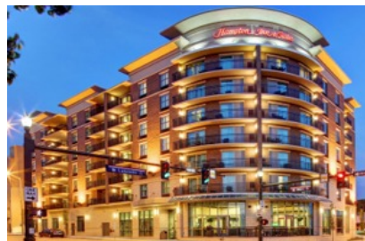
The new 137 Room Hampton Inn & Suites Baton Rouge Downtown
