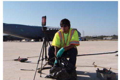
Lackland Air Force Base Apron Repair
