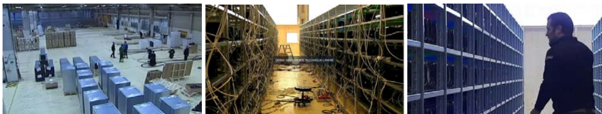
Figure 4: The KnC Miner Data Center in Sweden
