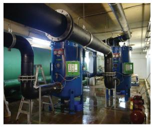
Sheraton Filter Room - Left = Sand Filters Right = Defender\* in 75% less space than sand filters
