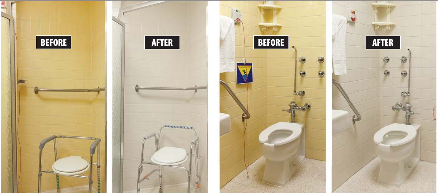
▲ Patient showers & bathrooms get a much needed renovation. Damaged tile & grout were repaired and permanently sealed.
