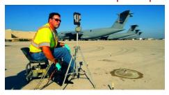
URETEK's engineers were able to stabilize and correct faulted and prematurely cracked airbase taxiways using URETEK's Deep Injection (UDI) Soil Stabilization process in 26 weekdays with minimal mission disruption.
