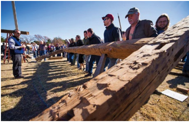
Timber frame barn assembly and raising
