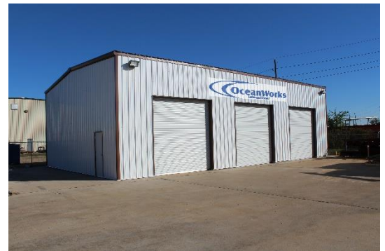
Figure 1 Completed Storage Facility
