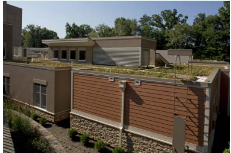
From green roofs to clerestory windows for extensive natural light indoors, the LEED Silver Certified Cohen Rosen House incorporates many green design features. Photography: Alain Jaramillo
