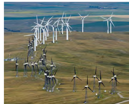
Southern Alberta wind farm Photo: Clive Schauptmeyer
