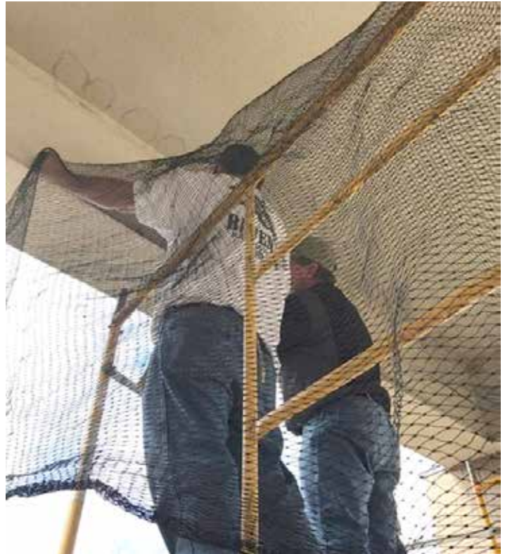
Raven Services installs Heavy Duty Bird Netting to exclude swallows from area.
