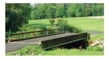
The QuickBridge<sup>®</sup> is an "off-the-shelf" solution for both temporary and permanent applications. The fixed-length The QuickBridge<sup>®</sup> can be built rapidly; most QuickBrldges are comprised of only two or three sections and can be installed with a minimal crew in under an hour. Its modular design also makes it suitable for a variety of applications, such as a footbridge or for site access.
