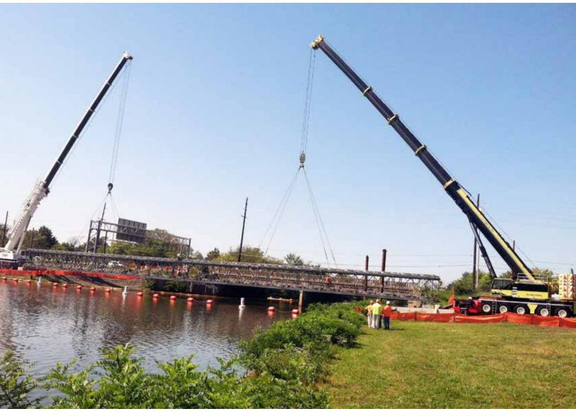
A 221 foot long pedestrian bridge in New Jersey being lifted into place using two cranes.
