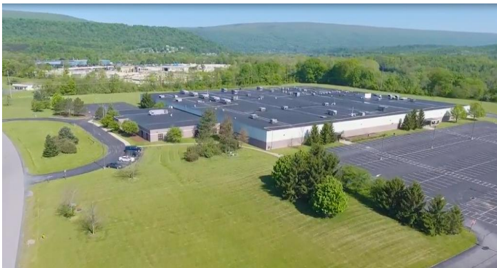
Aerial Shot of Mount Union, PA, Factory
