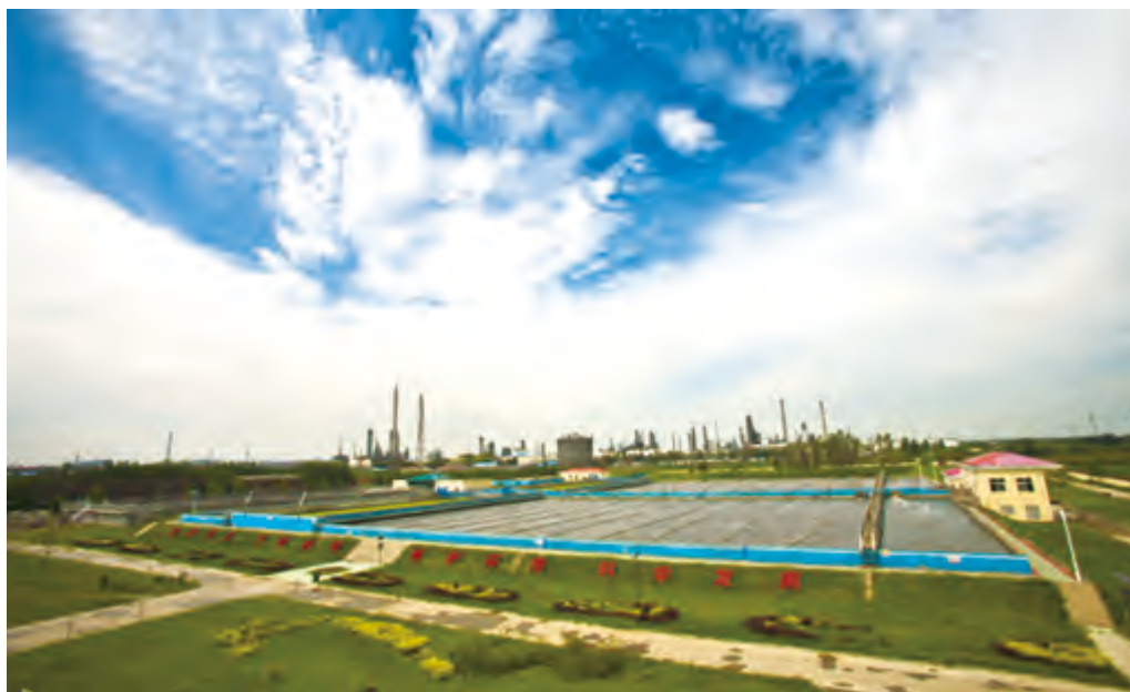
Water treatment facility managed and operated by a water management company in a third-tier Chinese city
