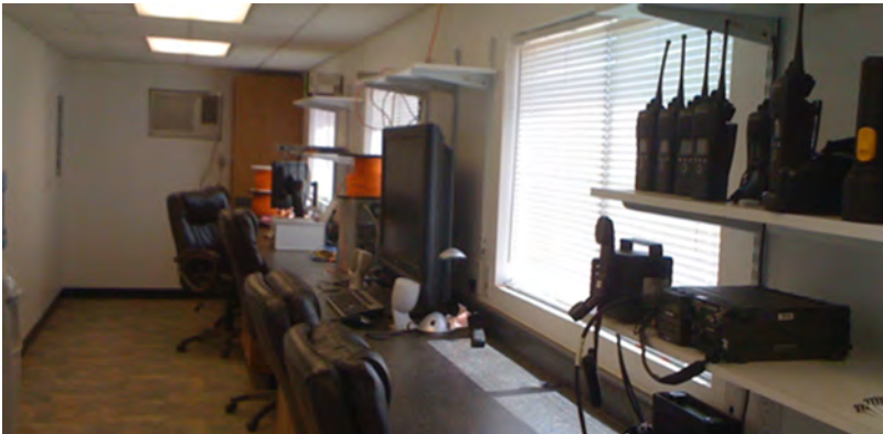
The ARC site control center.
