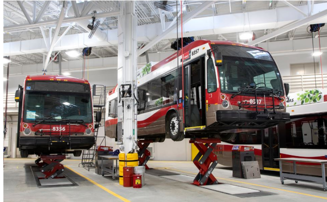
The facility has 36 service bays and 25 technicians capable of handling up to 470 transit buses. Photo courtesy of the City of Calgary.
