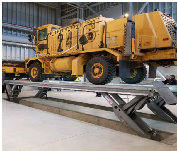
Large maintenance facilities increasingly turn to water-resistant vehicle lifting systems, such as the Stertil-Koni SKYLIFT Wash Bay, to clean their fleets
