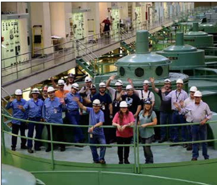
John Keys Pumping Plant, Grand Coulee Dam, Grand Coulee, Washington. Construction 1967-1974 (photograph: Reclamation, October 2019).
