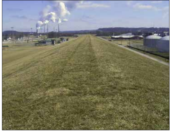
The Lawrenceburg levee system in Dearborn County, Indiana reduces flood risk from the Ohio River to the City of Lawrenceburg, Indiana (photograph: Army Corps, June 2010).
