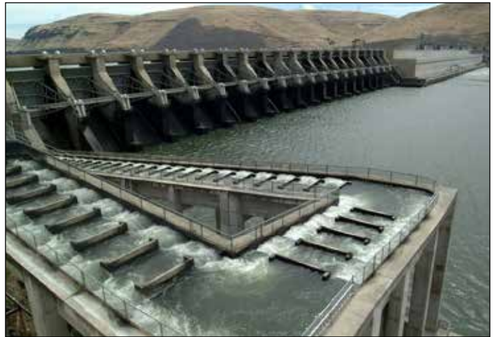
Fish ladder at John Day Lock and Dam, Columbia River near Rufus, Oregon (photograph: Army Corps, July 2002).
