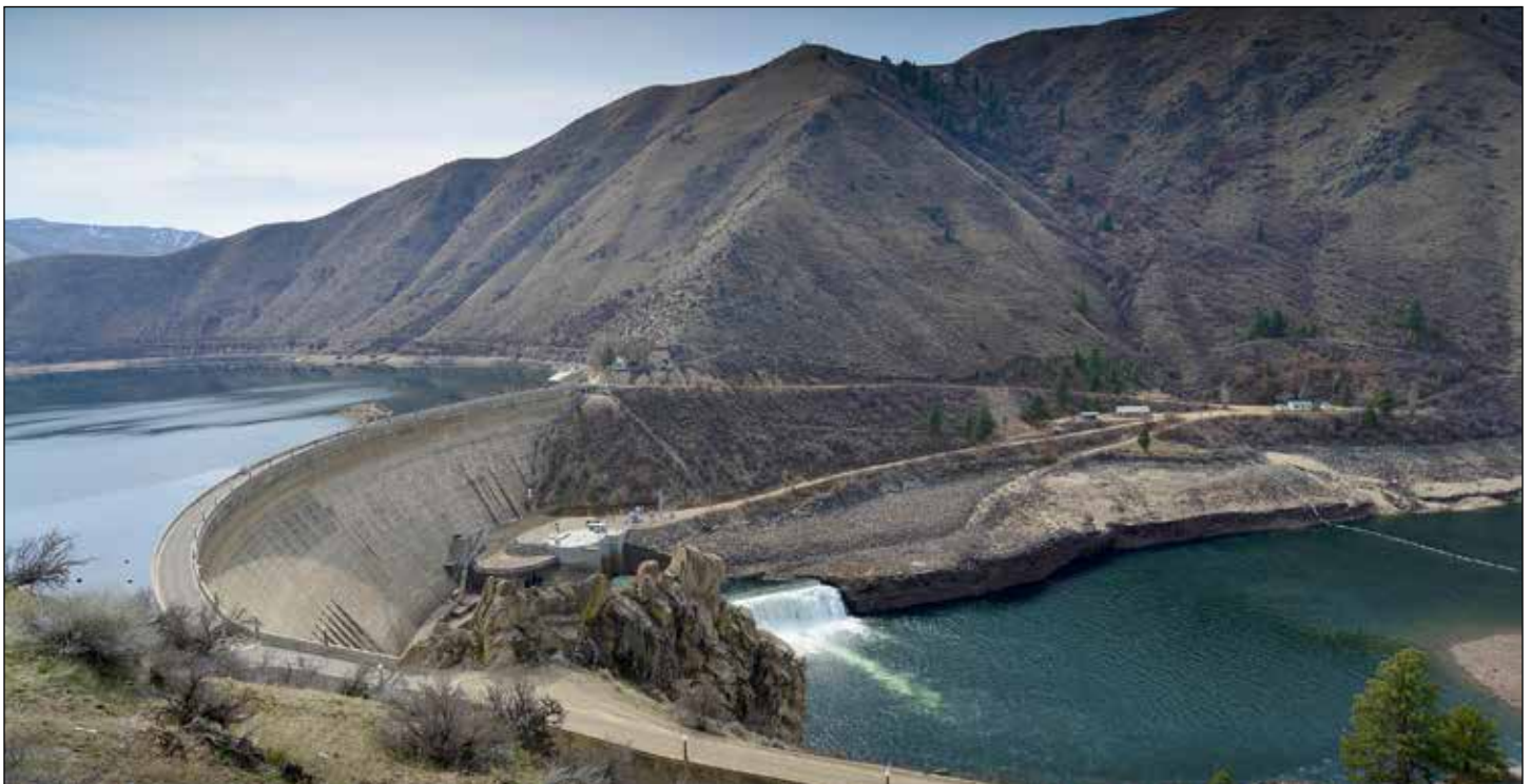
Arrowrock Dam, Idaho. Construction 1911-1915 (photograph: Reclamation, April 2013).
