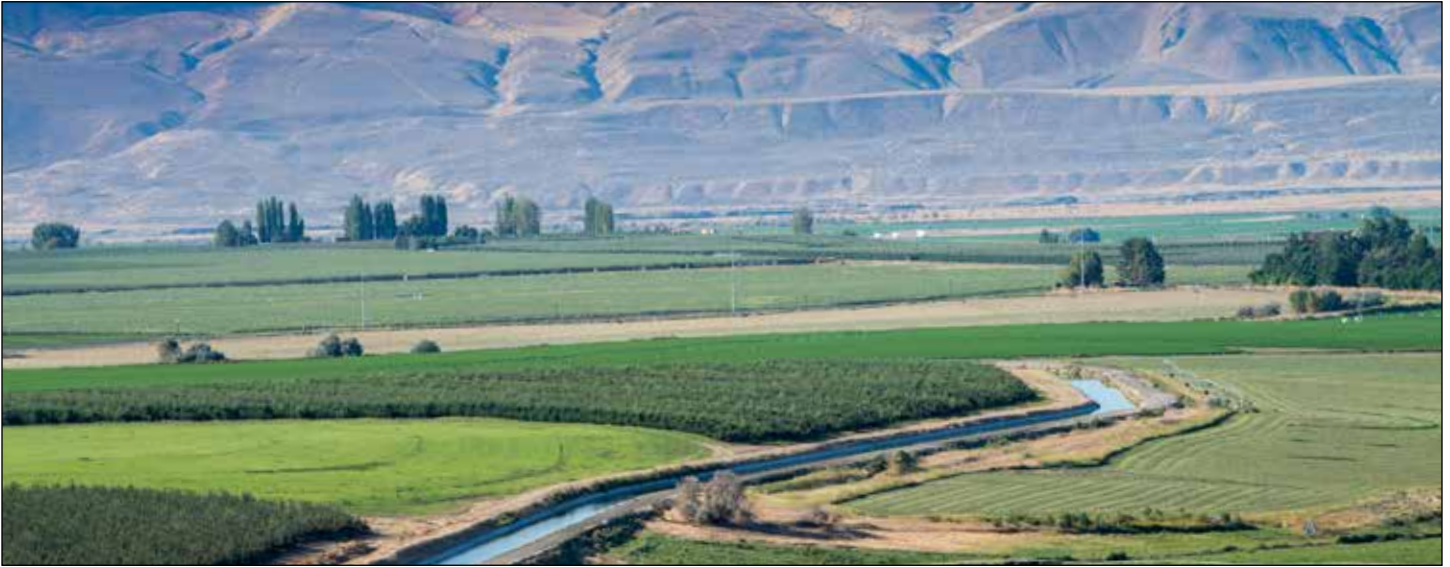
Potholes Canal, Columbia Basin Project, Washington (photograph: Reclamation, September 2018).
