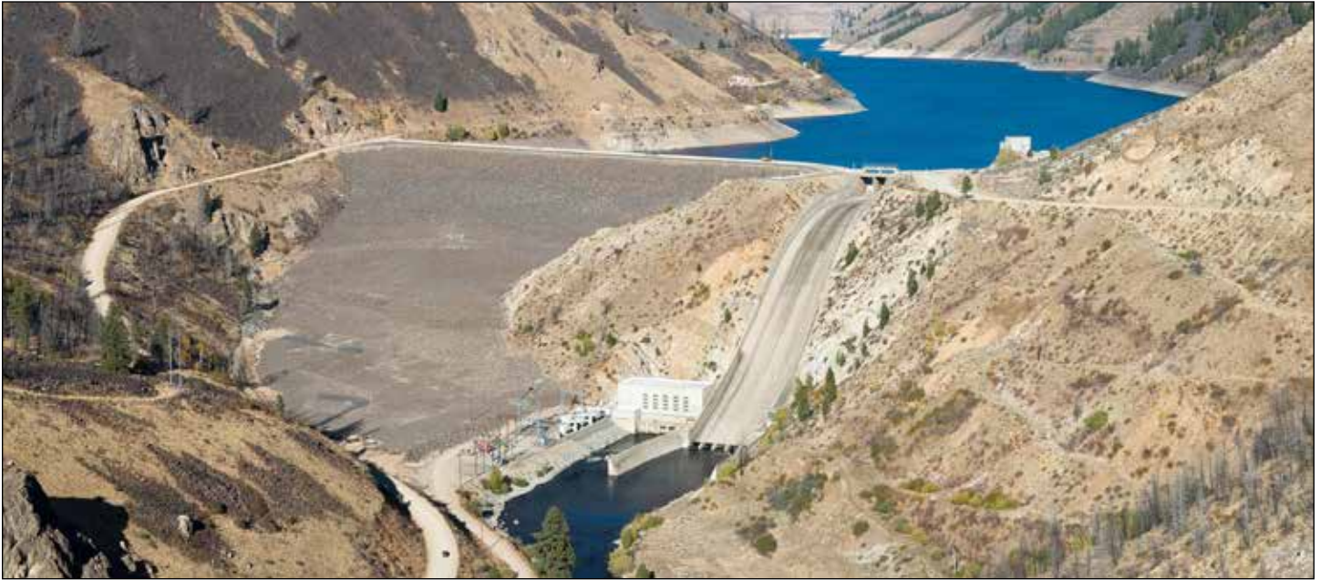
Anderson Ranch Dam, Idaho. Construction 1941-1950 (photograph: Reclamation, October 2018).
