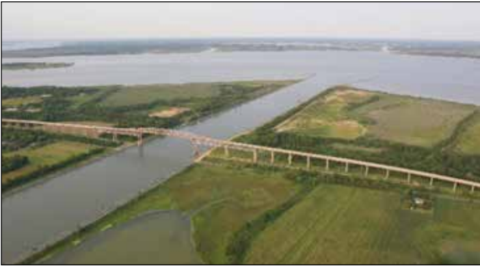
The Philadelphia District's Reedy Point Bridge at the Delaware River (Delaware Route 9), constructed in 1968, spans the Chesapeake and Delaware Canal connecting the Delaware River with the Chesapeake Bay in the states of Delaware and Maryland (photograph: Army Corps, August 2007).
