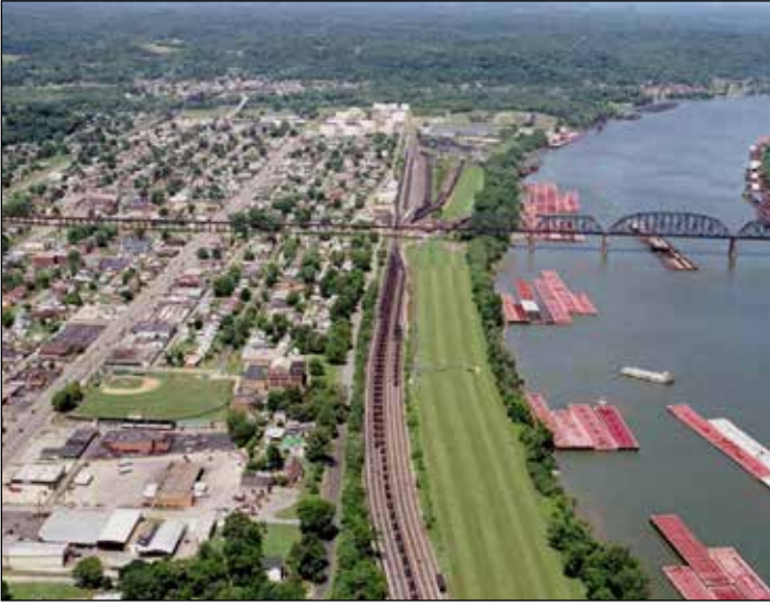
The Ceredo-Kenova Local Protection Project manages flood risk from the Ohio River and Big Sandy River to the cities of Kenova and Ceredo, Wayne County, West Virginia (photograph: Army Corps, circa 2001).
