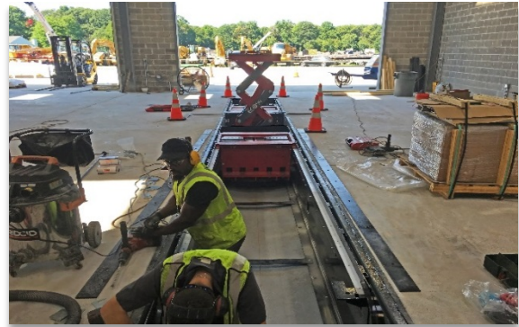
ECOLIFT features an ultra-shallow pit construction and arrives pre-assembled and tested
