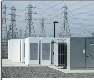
Figure 12: Energy Storage at a Substation
