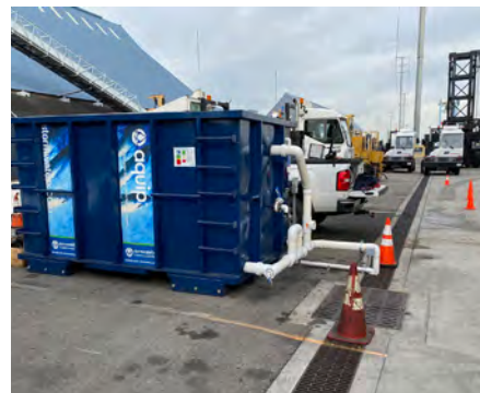
Trench drain with Frontline™ TDI filter inserts (not visible). AQUIP 50 downstream of TDI.
