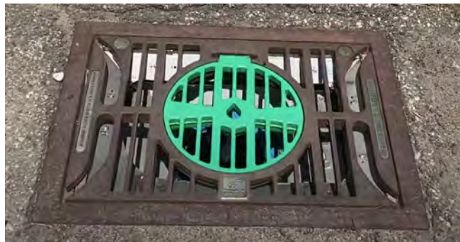
Frontline™ CBI under an existing catch basin grate
