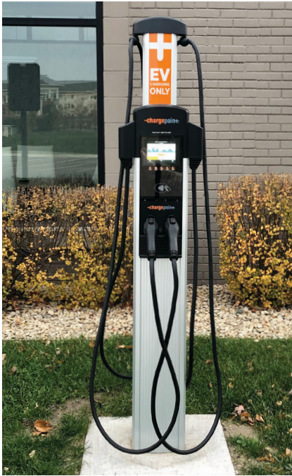
ChargePoint Dual Port Level 2 Charger
